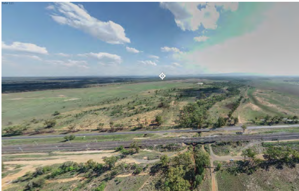
Figure 4.6 - Drone photograph looking south across along Charlevue Creek across the Capricorn Highway to the Project area (source: Magnetic South Pty Ltd)
