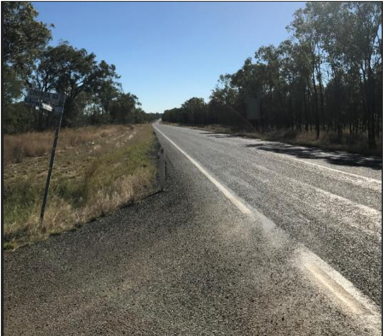
Figure 3-3 Capricorn Highway / Cooinda Road Intersection
