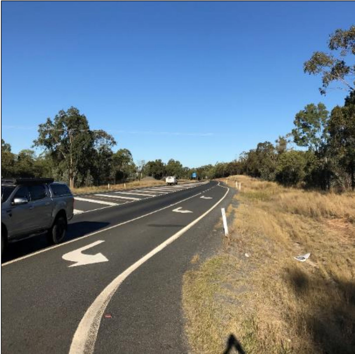
Figure 3-4 Capricorn Highway / Charlevue Road Intersection (facing east)
