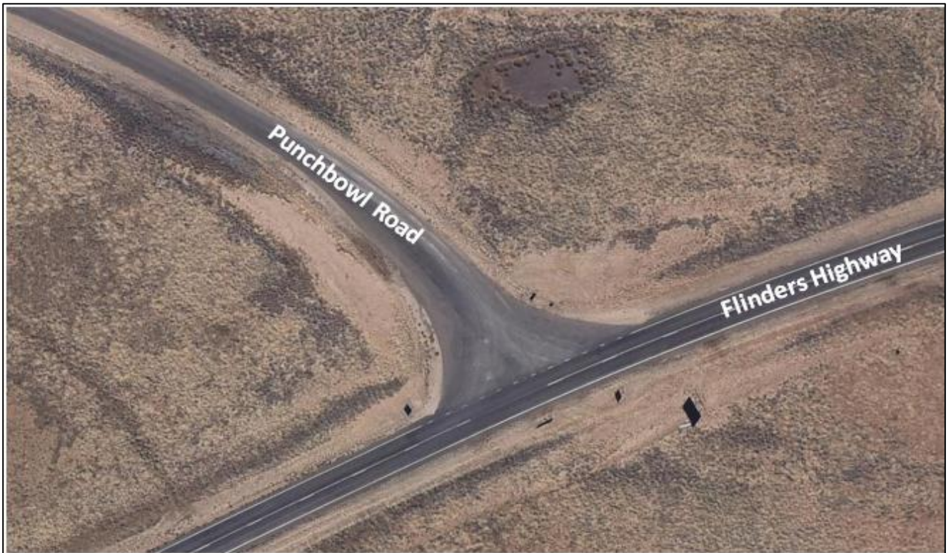
Figure 4.1 Flinders Highway / Punchbowl Road Aerial View
