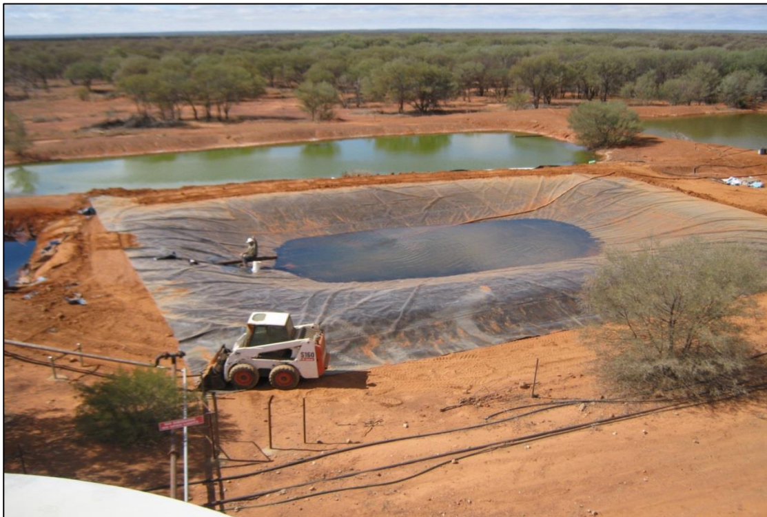
Figure 6 – Interceptor pond upgrade
