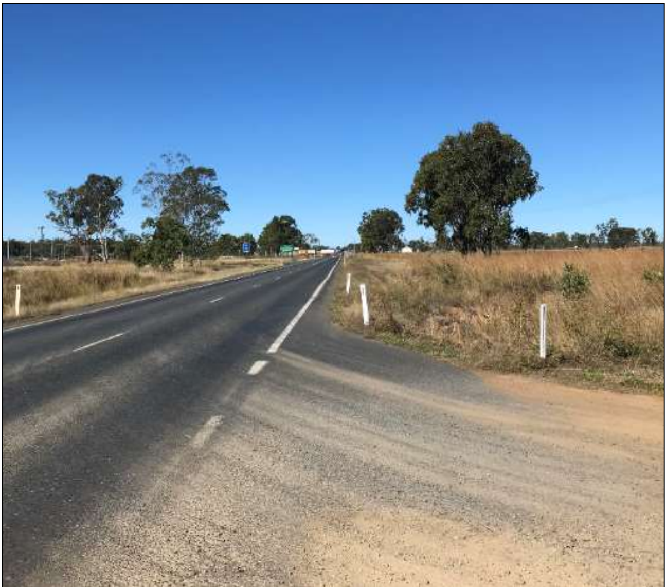
Figure 3-2 Capricorn Highway / Namoi Road Intersection (facing east)
