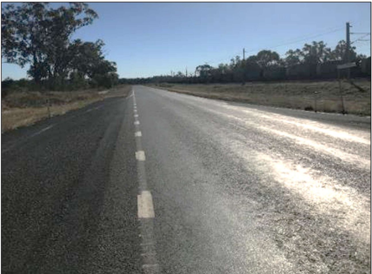
Figure 3-1 Typical section of Capricorn Highway (facing west)
