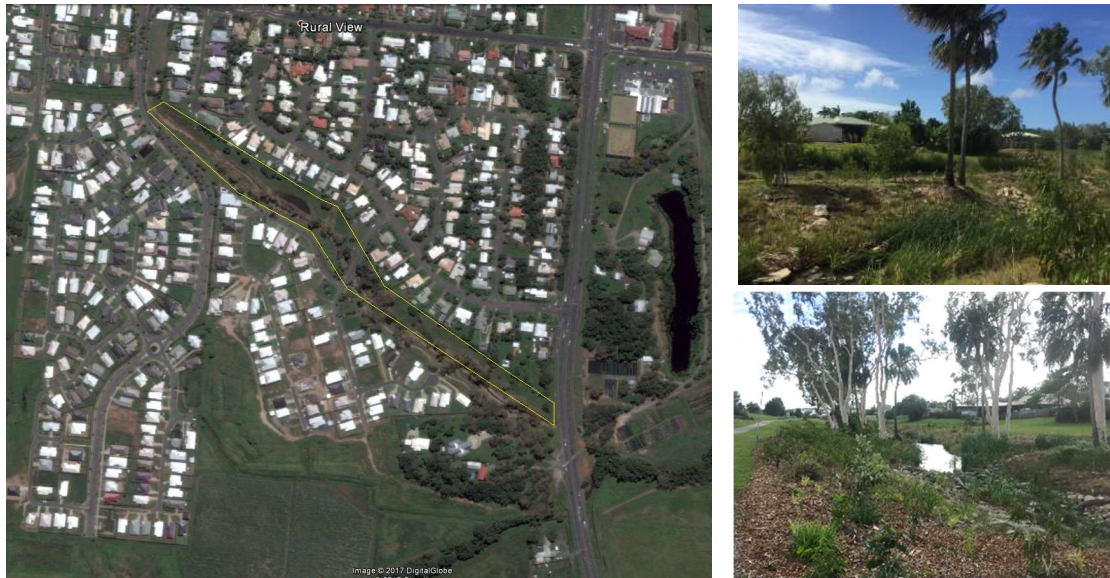
Figure 7. Site location (above) and finished works (right)
