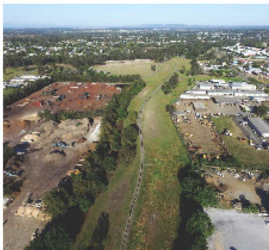
Overhead image of current site
