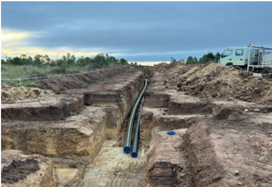
Photograph 1-1: Right of Way at pipe installation stage showing temporary disturbance.
