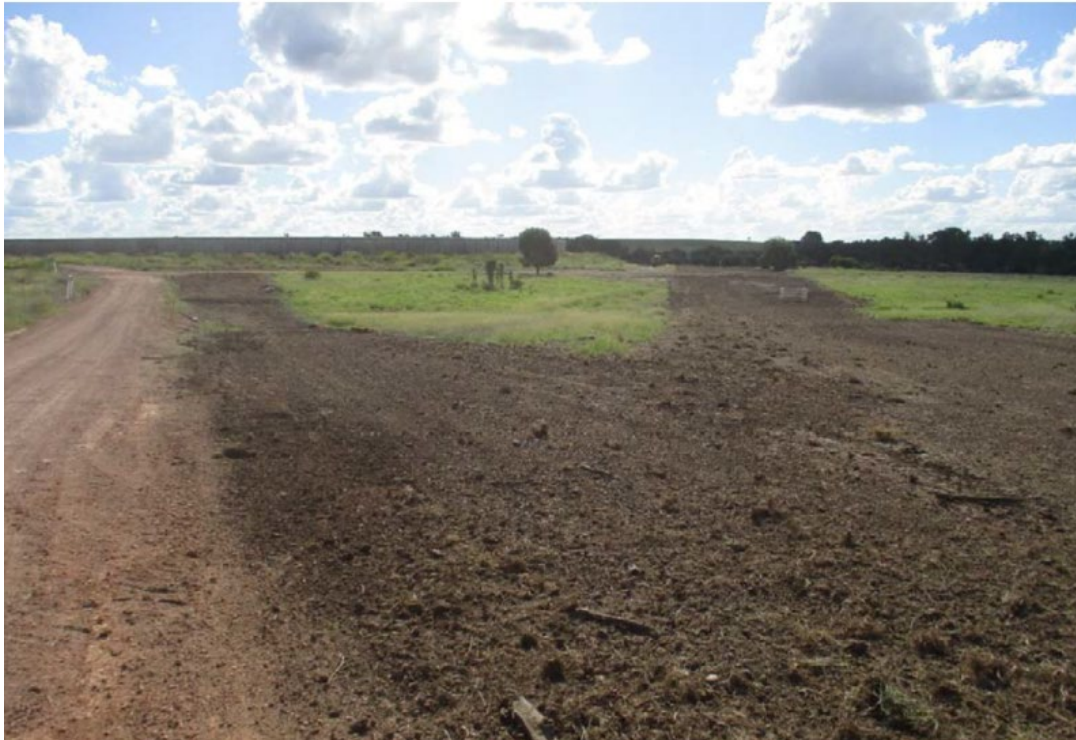
Photograph 1-2: Intersection of Two Right of Ways post construction showing no impedance of fauna dispersal.
