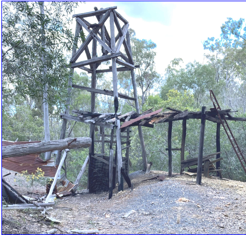
Plate 3: Old headstock with timber loading platform on right – small area ( 5m by 7m) of yellow grey mullock ( sample VJR03)
