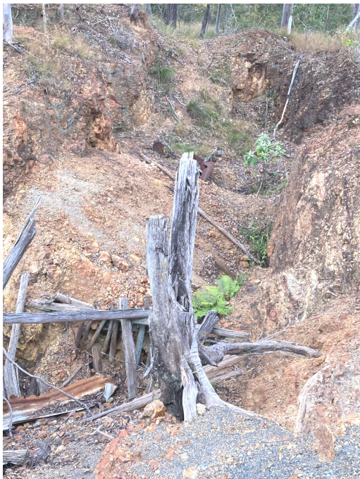
Plate 4 : Old pit near shaft – this is considered suitable to fill with waste rock (mullock) and as mining progresses. The pit is approximately 1,400 cubic metres in volume with solid rock (NAF) walls.
